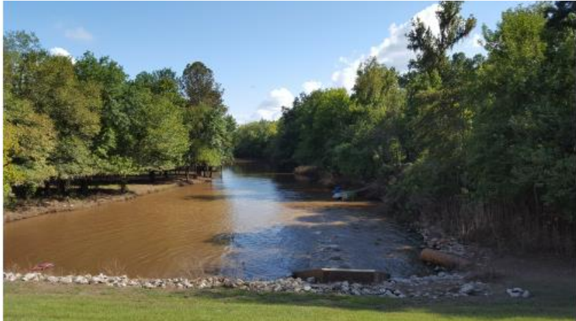
Bayou Ami-Borrow Pit ( 54" Culvert outlet in lower right)
